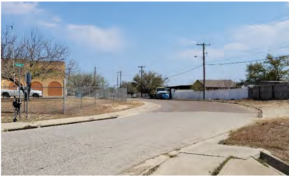
Looking at Wilson Road from US 59
